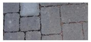
The joints on the right are full, where as the joints on the left require topping up with new joint aggregate.
